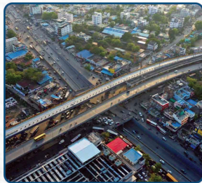
Biggest Junction LB Nagar Towards Vijayawada Highway
